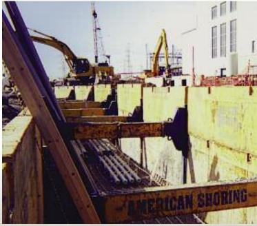
Shown above is an installation of a 23'D x 12'H x 10'W precast concrete box culvert using Mega Rolling Strut™ Slide Rail with a clearance of 16' under the cross brace for the NYCDEP in Brooklyn, NY.
