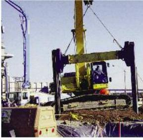
Shown above is an installation of duct banks using our Rolling Strut™ Slide Rail System for Public Service Electric & Gas at Linden, New Jersey generating plant expansion project.
